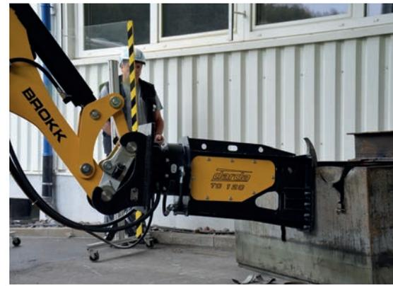
The new TC120 tank cutter, combines with an electric Brokk demolition machine to tackle a steel tank
